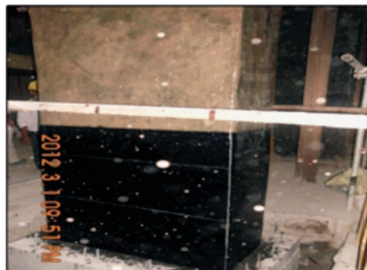
Figure 11. Strengthened wall and column (Courtesy of DPWH Central Office)
