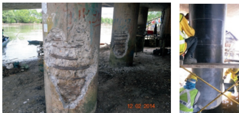
Figure 9. Column before and after Carbon FRP application (Courtesy of SIKA Philippines)
