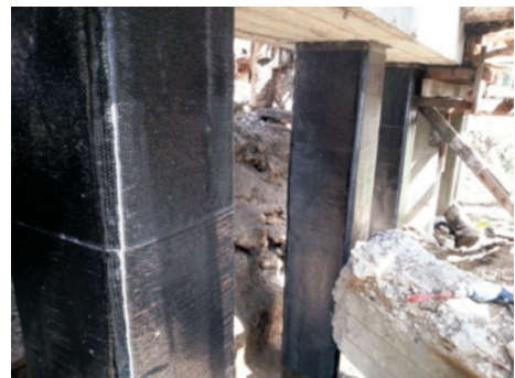
Figure 8. Column before and after Carbon FRP application (Courtesy of SIKA Philippines)
