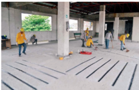
Figure 10. Strengthening of Montelibano Hospital (Courtesy of SIKA Philippines)
