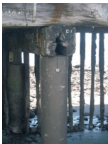
Figure 4. Hollow FRP pipe piles (Courtesy of BAC Tech. Pty. Ltd., Queensland, Australia)
