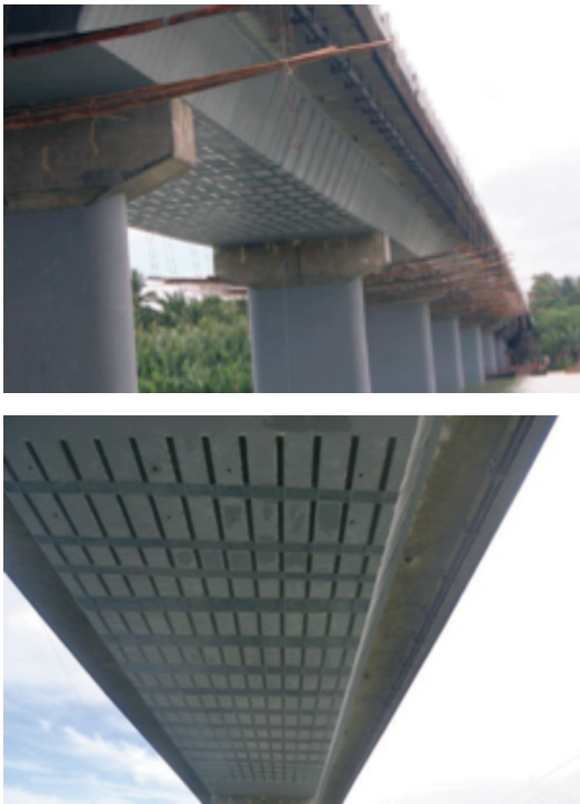
Figure 7. Strengthened Bago Bridge in Negros Occidental (Courtesy of SIKA Philippines)
